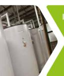
Incoming water is pre-heated using the waste water reducing energy consumption across the entire site
