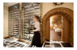
The Towers are all 3 metres high by 1.5 wide. Two have glass sides all round and three have stainless steel backs, to go against the wall. Four are connected to remote refrigeration, whilst the fifth uses its integral system.
